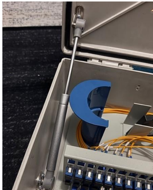
Figure 9. Hydraulic Actuator Installation
